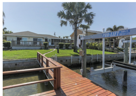
The dock has been rebuilt and new wrapped pilings installed.
